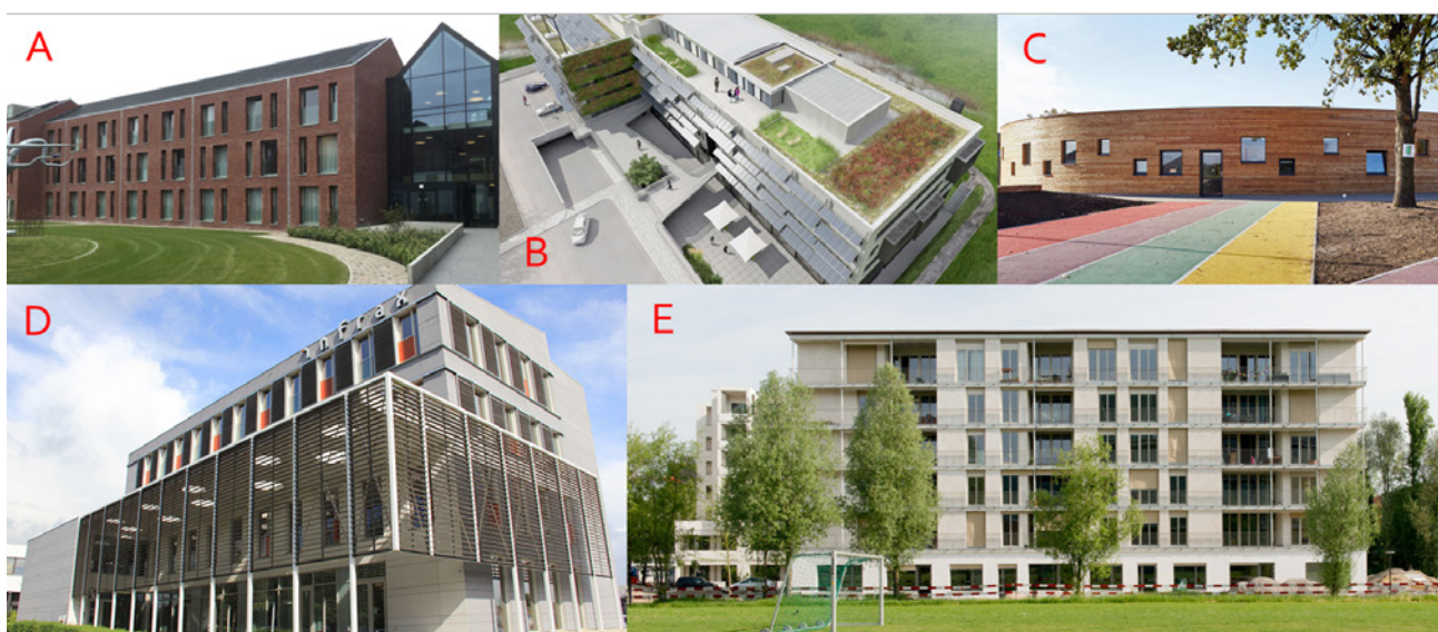
Figure 3. hybridGEOTABS demo buildings: A) TerPotterie, Bruges B) Solarwind, Windhof C) Libeznice primary school, D) Infrac building, Dilbeek E) Haus M, Zurich. Image credits: hybridGEOTABS project ( www.hybridgeotabs.eu )
